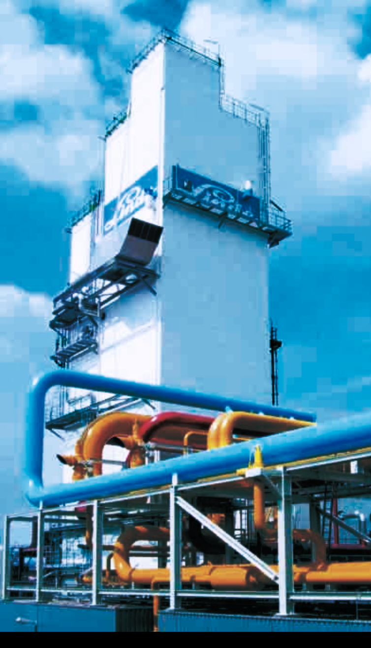
Linde installs largest air separation unit in Austria.
