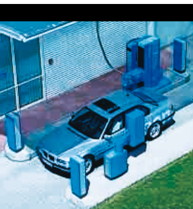
The hydrogen fueling station at Munich Airport gives a sneak preview of the new station planned for Berlin. Linde will supply the liquid hydrogen (LH 2 ), cryogenic fuel tank, pump, compressor station and peripheral fueling equipment. Both liquid and gaseous re-fueling equipment will be installed.
